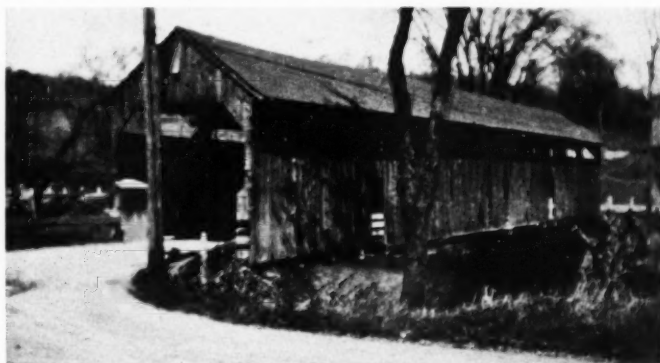
Burkeville Covered Bridge, over South River, Conway, Mass.
